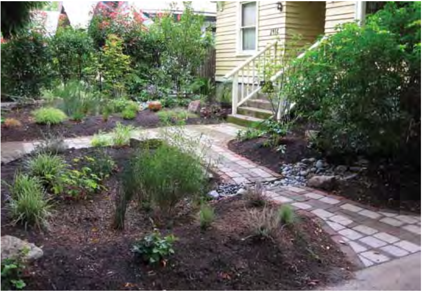
Figure 11: Using a rock-lined trench to convey water across a walkway (Photo: Portland Bureau of Environmental Services [BES])
