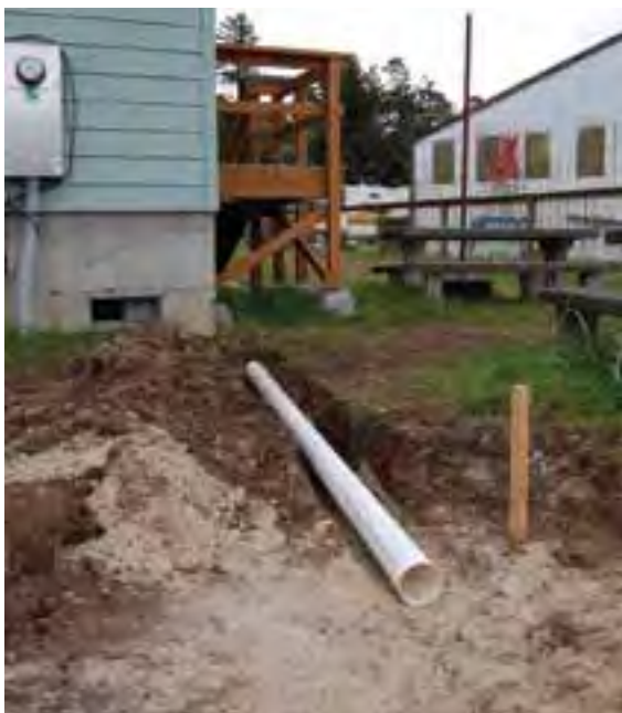
Figure 22: Four-inch ABS pipes here will convey water from this building into a rain garden. Pipes like these must be graded to drop about 1 inch for every 10 feet so water flows away from the building but does not build up too much velocity by the time it arrives in the rain garden. (Photo: Robert Emanuel, OSU)
